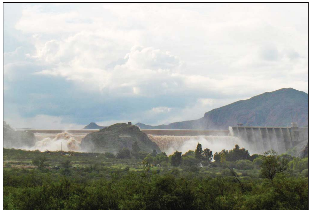
Las Virgenes dam, Mexico, September, 2008: The reservoir was vastly overfull with water and dam operators had to spill excess water to prevent the dam from breaching. Note the frothing water on the left spillway.
