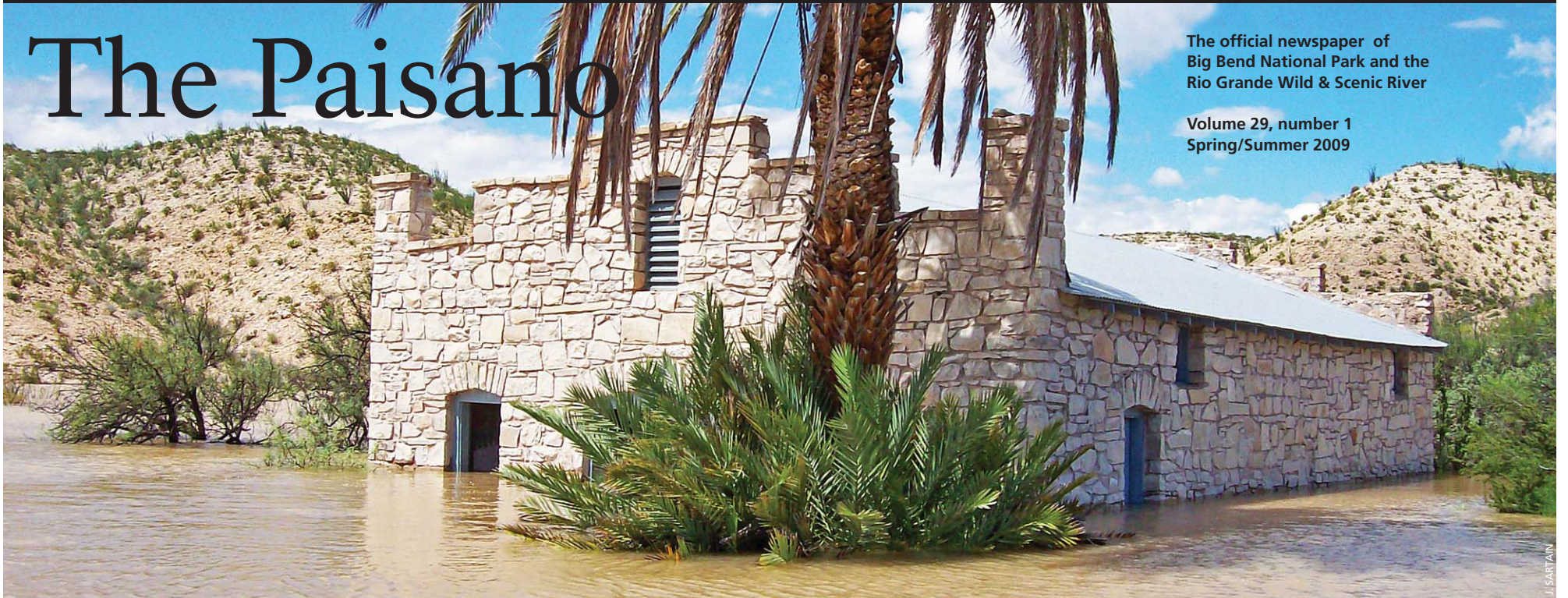
Floodwaters back up into the Langford Store ruin
